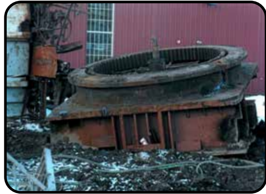
Pivot ring and base January 28, 2023. It was a cast steel piece about 4-6 inches thick and close to 12 inches high.
