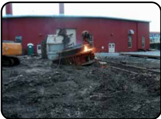
Torching the ring gear into pieces the trackhoe could pick up. January 31, 2023
