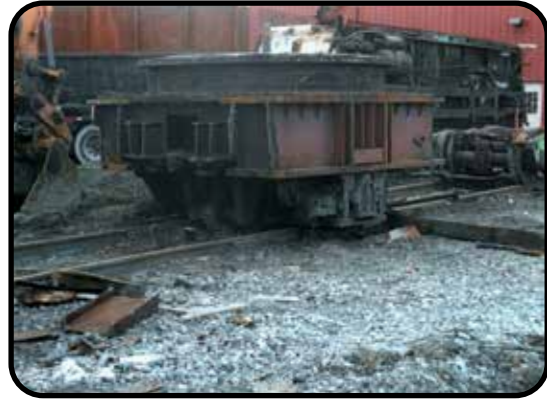
Center power truck showing gears used to transmit power to end power truck gears (right side of photo). January 24, 2023
