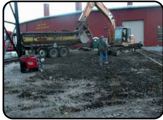
Last piece of base structure loaded on the truck. February 6, 2023
