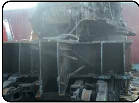
End frame of crane cut off revealing the heavy under crane frame. January 10, 2023
